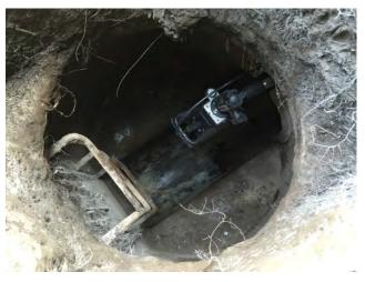
Figure 2-9. Area-Velocity Meter Installation Setup in Sewer (Flow-Tronic)
