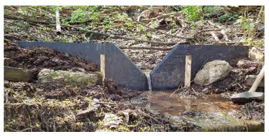
Figure 2-5. V-notch Weir (PWSA)
