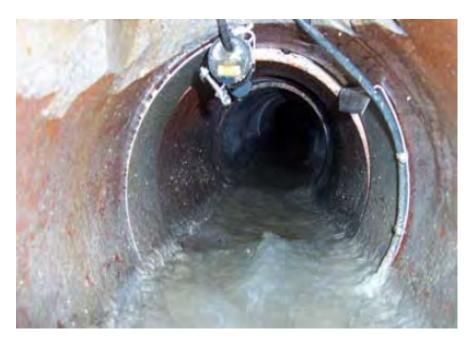
Figure 2-22. In-sewer Monitoring with Area-Velocity Flow Meter (ALCOSAN)
