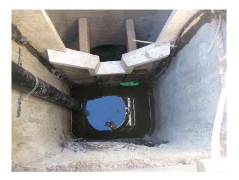
Figure 2-21. Weir Installed in Manhole for in-GSI Monitoring of Outflow. (CVC) Level sensor is mounted on upstream side of weir.
