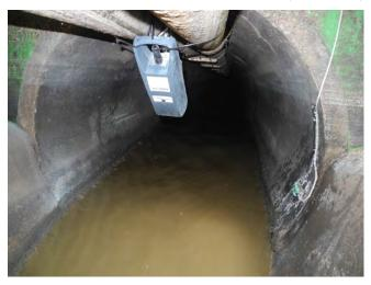
Figure 2-10. Example showing monitor installed at the top of the pipe
