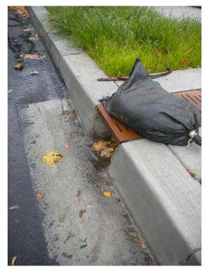
Figure 2-2. Water bypassing the trench drain inlet due to an improperly constructed concrete apron
