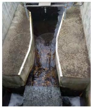
Figure 2-6. Parshall Flume (www.openchannelflow.com)
