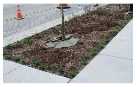
Figure 2-17. Plants near GSI Edge Stormwater planter in which the plants have been installed too close to the edges
