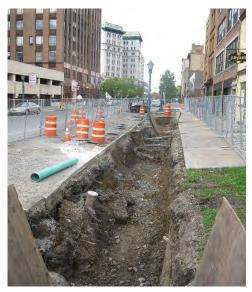
Figure 2-2. ROW Construction Site Safety fencing and drums help to create a barrier for this infiltration trench
