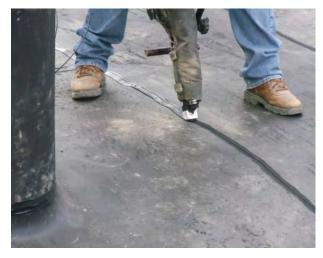
Figure 2-23. Impermeable Liner Liners used for constructed wetlands must be properly sealed and pass all specified tests
