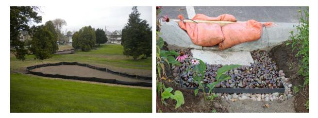
Figure 2-3. Silt Fence Around GSI Silt fence can help protect bioretention areas until contributing areas are stabilized or until vegetation has been planted/established
