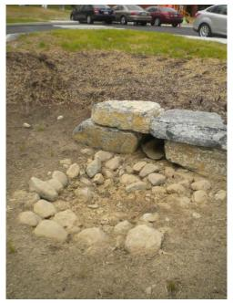
ay restore the systemFigure 2-7. Sediment in Bioretention Areafunctionality. InspectionsExample of a bioretention area that has beenfollowing heavy rainfallsimpacted by sediment-laden runoff
