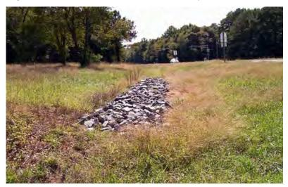
Figure 2-10. Surface Flow Infiltration Trench Infiltration trench with stone surface (source: <u>Maryland Department of Transportation</u>)
