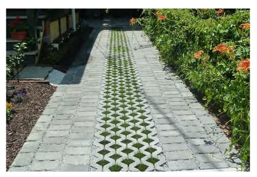
Figure 2-15. Open Grid Pavers Open grid pavers in Philadelphia, PA (source: <u>Philadelphia Water Department)</u>
