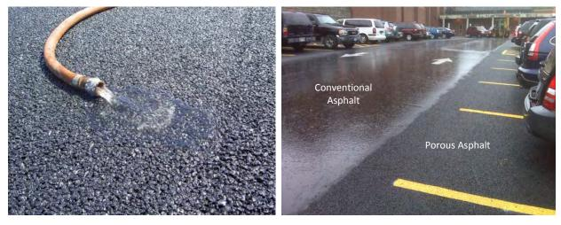
Figure 2-12. Porous Asphalt Surfaces
