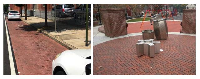
**Figure 2-14. Permeable Pavers** *Permeable pavers in a parking lane and in a pedestrian plaza*
