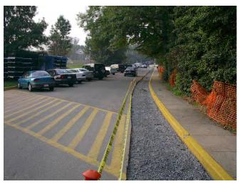
**Figure 2-8. Infiltration Trench** Infiltration Trench along curb under the roadway
