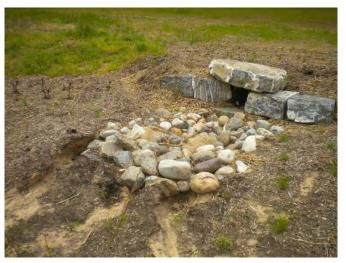
**Figure 2-3. Erosion in Bioretention Area** Erosion damage in a bioretention area with inadequate energy dissipation and lack of vegetative growth
