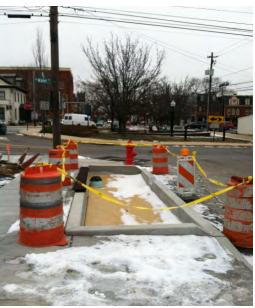
**Figure 2-15. Planter in Winter** "Winterized" stormwater planter in which the planting was delayed until the spring with safety drums and caution tape to protect it
