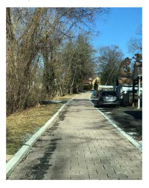
Figure 2-14. Excess Gravel on Permeable Pavers Permeable pavers in a residential alley require vacuuming to remove excess gravel and organic debris from adjacent properties.
