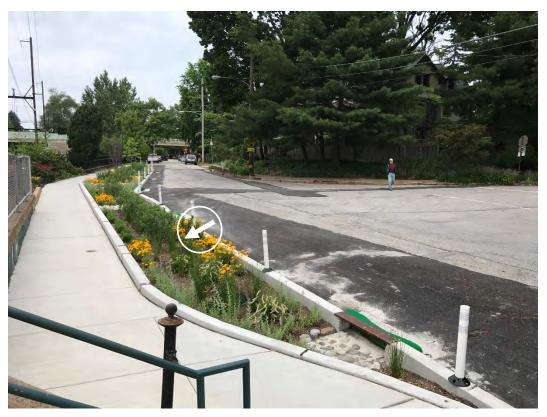
**Figure 2-3. ROW Curb Extension** Example of a vegetated curb extension (indicated by arrow) in the public right-of-way in front of Sedgwick Station located in Philadelphia, PA and implemented by the Philadelphia Water Department
