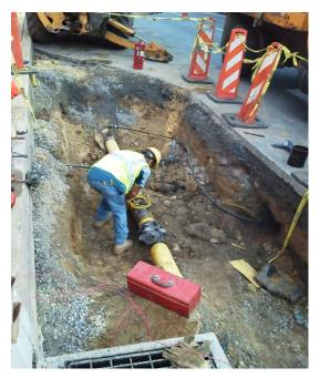
Figure 2-8. Utility Protection At this vegetated curb extension installation, a contractor ensures that a previously unknown existing gas line is sufficiently protected from potential damage by the GSI facility
