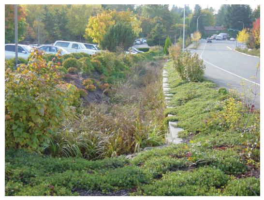
Figure 2-3. Vegetated Swale Bioswale between a road and parking area
