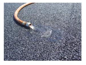
**Figure 2-11. Porous Asphalt** The surface of porous asphalt requires regular vacuum sweeping to maintain surface porosity.
