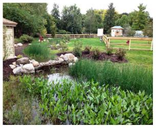
Figure 2-24. Constructed Stormwater Wetlands Constructed stormwater wetlands must be graded to conform to design drawings to achieve optimal performance
