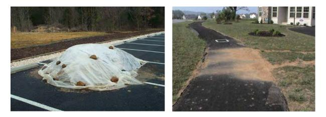
Figure 2-13. Material Storage and Sediment on Permeable Pavements Permeable pavements should never be used for particulate material storage and adjacent vegetated areas should be regularly maintained to prevent erosion and sediment run on.
