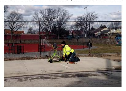
Figure 2-9. Pipe Condition Inspection An inspector feeds a video camera through a cleanout and perforated distribution pipe within an infiltration trench, while reviewing pipe conditions on a video monitor.
