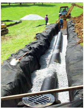
**Figure 2-9. Infiltration Trench** *Infiltration trench in turf grass*
