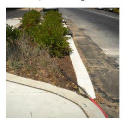
Figure 2-6. Example of Vegetation Watering A temporary irrigation hose in this vegetated system helps ensure proper watering during plant establishment.
