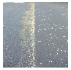
Figure 2-1. Debris on Porous Asphalt Example of porous asphalt starting to clog along its interface with conventional asphalt due to vegetation debris; <u>Sunnycrest Arena</u> in Syracuse, NY; implemented by Onondaga County
