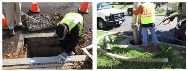
**Figure 2-2. Collection System Maintenance** *Regular conveyance system maintenance may be completed by hand or with a vactor truck.*
