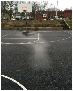
Figure 2-15. Puddles on Porous Asphalt Surface puddles on a porous asphalt basketball court indicate the pavement is partially clogged by run-on and requires corrective action such as power washing and high-suction vacuuming.
