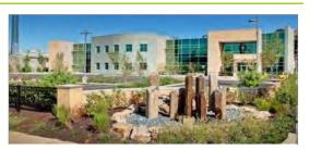
Figure 6-10: ALCOSAN's CS&T Building parking lot uses a rain garden and bio-swale to capture and infiltrate stormwater
