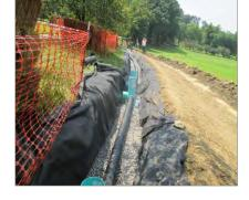
Figure 6-9: Infiltration trenches and berms have been installed to reduce hillside erosion, converting lawns to meadows, and vegetative buffers in Pittsburgh's Schenley Park.
