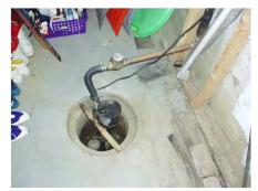
Figure 6-5: Sump pump disconnection from sanitary sewer
