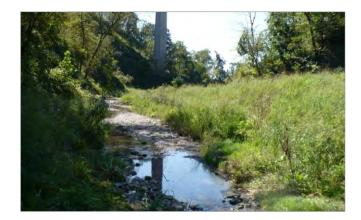
Figure 6-6: Jack's Run stream was re-routed out of the combined sewer system and restored
