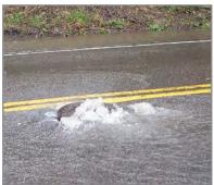
Figure 6-8: Sanitary Sewer Overflow Caused by Excessive Inflow and Infiltration
