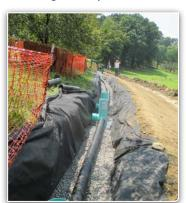
Infiltration trenches and berms have been installed to reduce hillside erosion, converting lawns to meadows, and vegetative buffers in Pittsburgh's Schenley Park.
