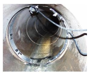
Figure 4-9: Looking upstream along a sewer pipe with installed flow monitoring equipment
