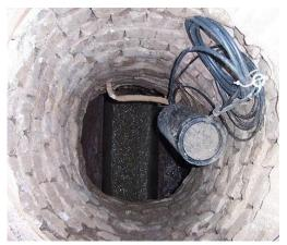
Figure 4-8: Looking down at flow monitoring equipment installed within a sewer manhole
