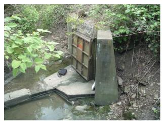
Figure 4-15: Typical example of a flap gate used to prevent stream flow from entering the ALCOSAN system
