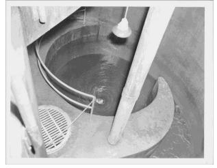
Figure 4-14: Typical example of a vortex drop-shaft used to convey flow to the deep tunnel system
