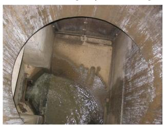
Figure 3-4: Interior view of an ALCOSAN regulator structure diverting flow for treatment
