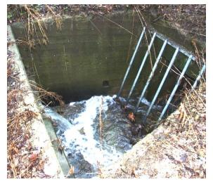
Figure 3-8: A creek along Spring Garden Avenue is culverted and becomes the Spring Garden combined trunk sewer serving Reserve Township and the City of Pittsburgh.
