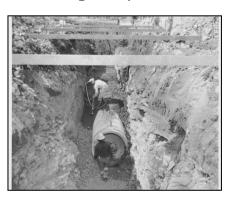
Figure 1-3: Construction of the shallow cut portions of the ALCOSAN interceptor system
