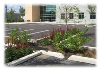
Figure A-1: Example of Curb Cut-out with Bio-Swale at ALCOSAN Customer Service & Training Building
