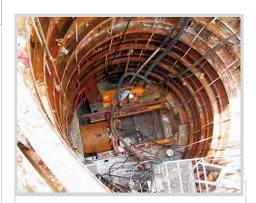
Much of the new consolidation sewers in the UM Basin Facilities Plan will be constructed using trenchless technology like microtunneling (pictured above) to minimize surface disruption
