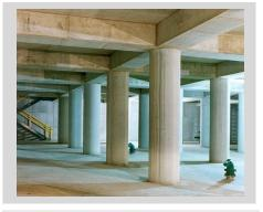
The basin storage facility above, located in Van Buren Township, Michigan, is an example of one the types of control of technologies being evaluated to control overflows in the LOGR Basin. This 1.3-MG storage basin is used to balance sewage flows between available capacities in three regional sewer systems. It is covered by earth and features green storm water management practices including a bioswale and storm water reuse to flush the basin after use.
