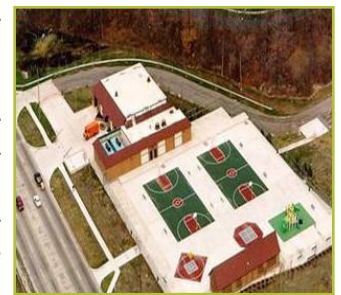
Underground Storage Tank
