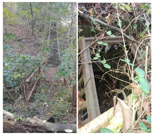
**Figure 9**. Bridge over existing channel and inlet structure at Potential Inflow Location CC-31
