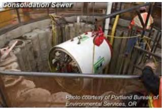
**Main tunnels** are planned to be 16 to 18 feet in finished diameter and will be constructed an average of 150 feet below ground. They will primarily be constructed using large tunnel boring machines (TBMs) that will be lowered from the surface and later retrieved via construction shafts.
