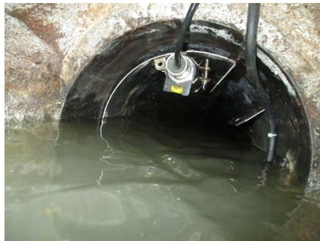
Figure 2-8. Area Velocity Meter Installation Setup in Sewer
