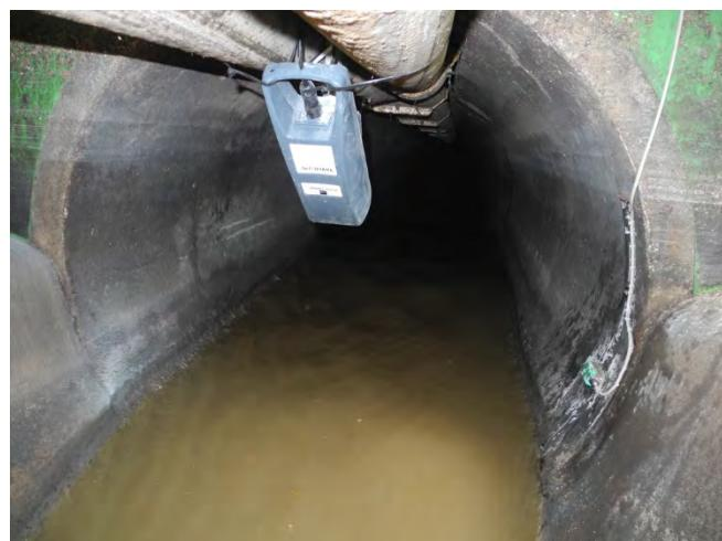
Figure 2-10. Example showing monitor installed at the top of the pipe
