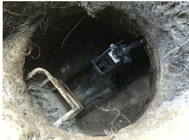
Figure 2-9. Area-Velocity Meter Installation Setup in Sewer
