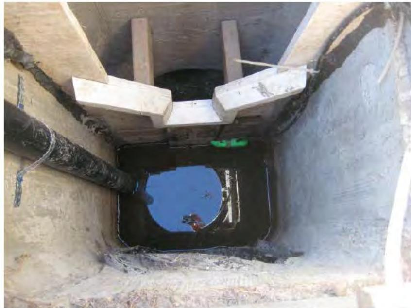
Figure 2-21. Weir Installed in Manhole for in-GSI Monitoring of Outflow. (CVC)
