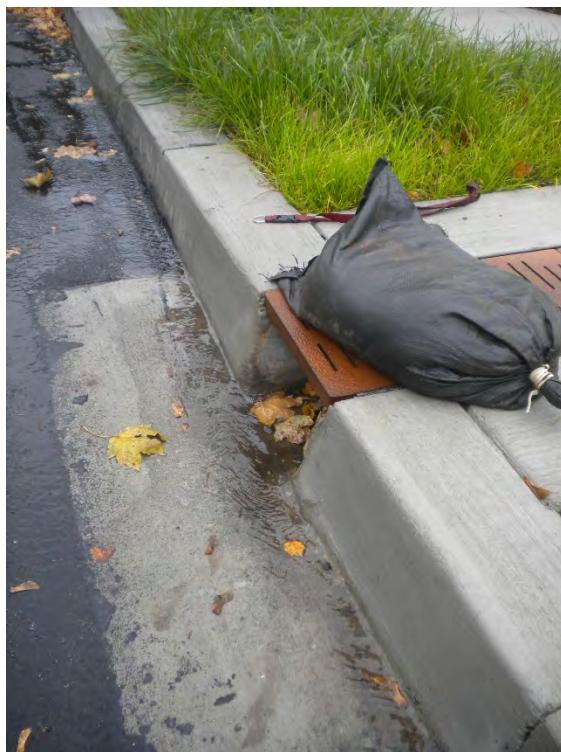
Figure 2-2. Water bypassing the trench drain inlet due to an improperly constructed concrete apron
