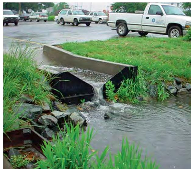
Figure 2-14. Channel and Weir Serving as a Sheet Flow Concentrator (Gwinnett County)
