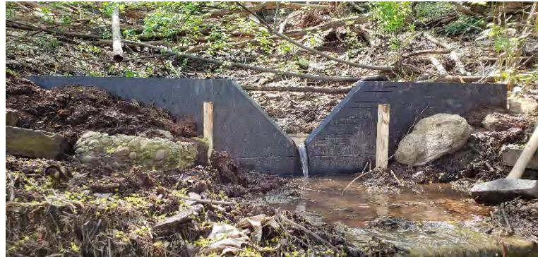
Figure 2-5. V-notch Weir (PWSA)
