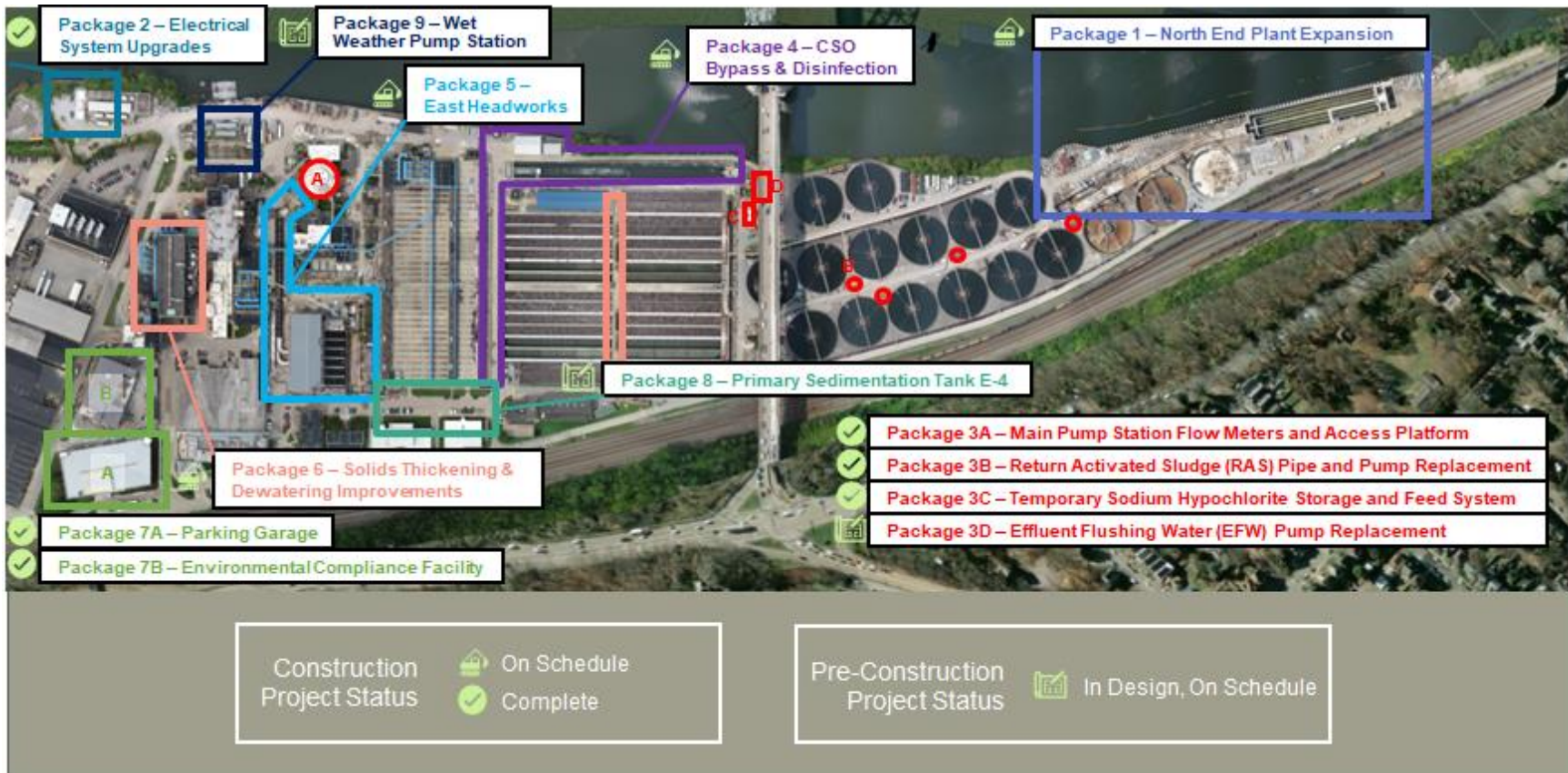
Figure 1: Wastewater Treatment Plant Expansion Construction Progress
