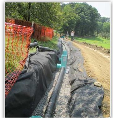
*Infiltration trenches and berms have been installed to reduce hillside erosion, converting lawns to meadows, and vegetative buffers in Pittsburgh’s Schenley Park.*
