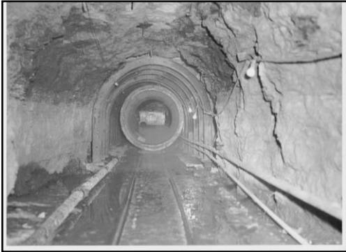
**Figure 1-4: Construction of the deep tunnel portions of the ALCOSAN interceptor system**
