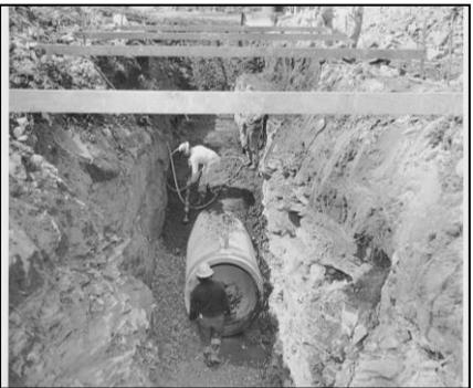
**Figure 1-3: Construction of the shallow cut portions of the ALCOSAN interceptor system**
