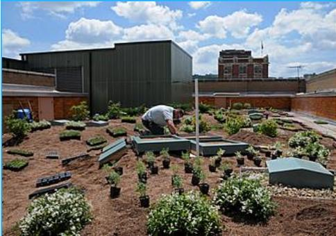
Figure A-6: Ongoing maintenance at the Allegheny County office building's green roof
