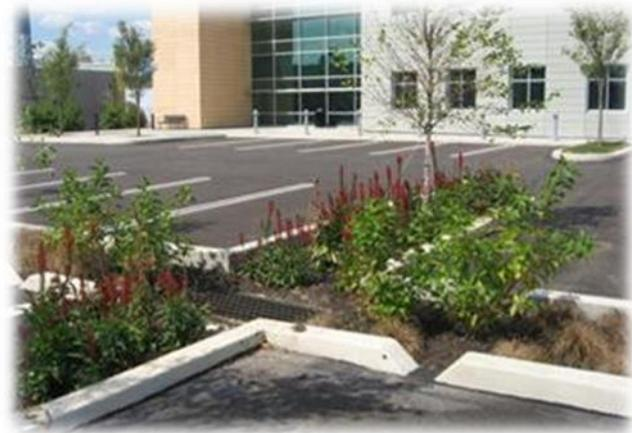
*Figure A-1: Example of Curb Cut-out with Bio-Swale at ALCOSAN Customer Service & Training Building*
