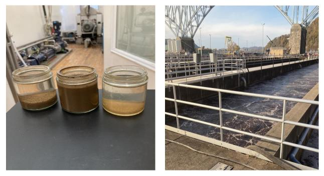
Figure 1.0 is a visual representation of the feed, thickened sludge, and centrate liquor produced by the ALSYS G3-75 thickening unit. Figure 2.0 is a visual representation of the feed from the aeration basin
