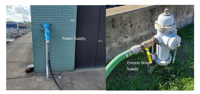
Figures 5 and 6. Thickener skid 480V power supply connection and process water connection.
