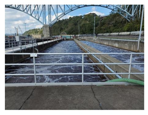
Figure 4. WAS feed hose pulling out of EA-4 Pass-1.
