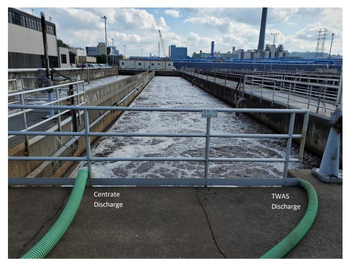
Figure 4. Centrate and TWAS hoses discharging into EA-4 Pass-2.
