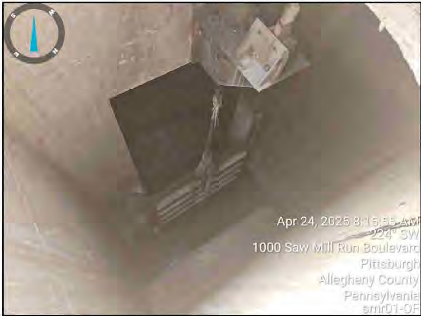
EXISTING WEIR GATE S-01A OVERFLOW CHAMBER
