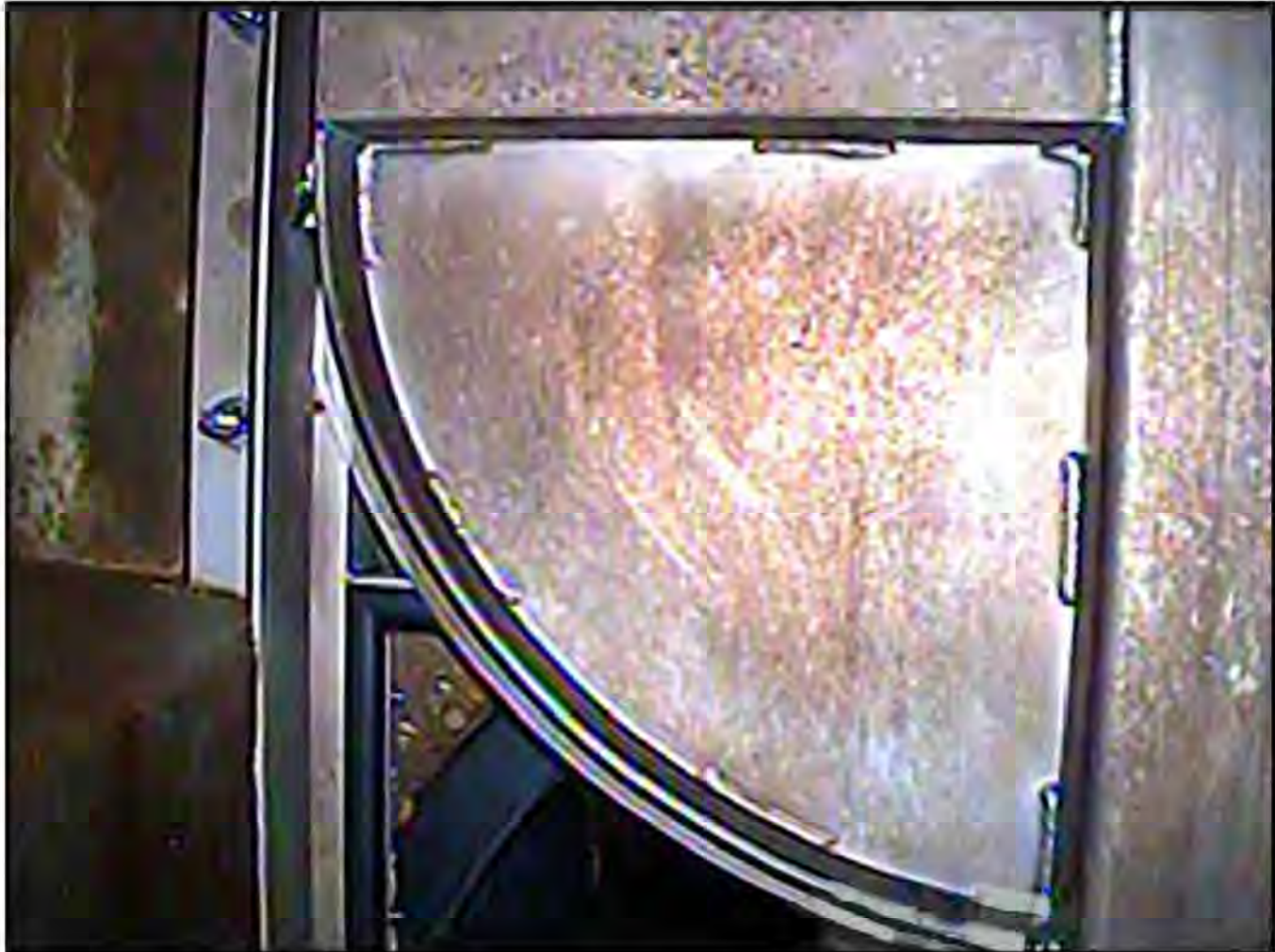
EXAMPLE EXISTING ROUND BOTTOM FABRICATED SLUICE GATE
