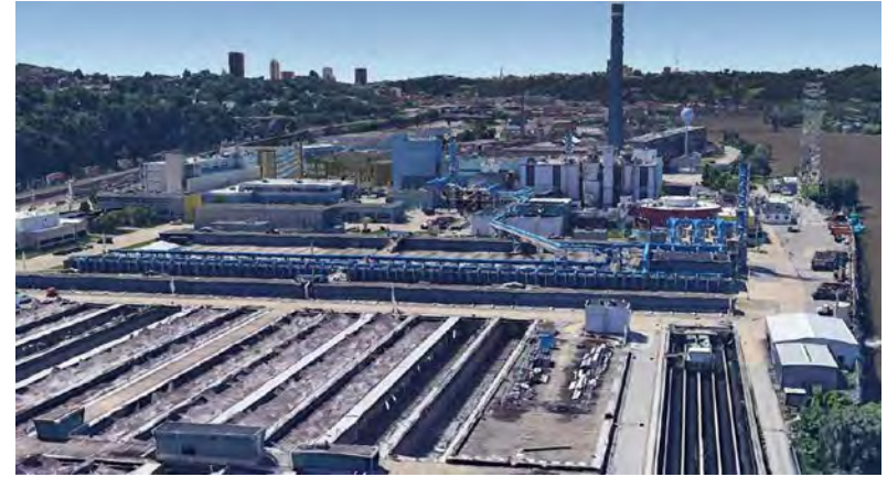
View from the McKees Rocks Bridge
