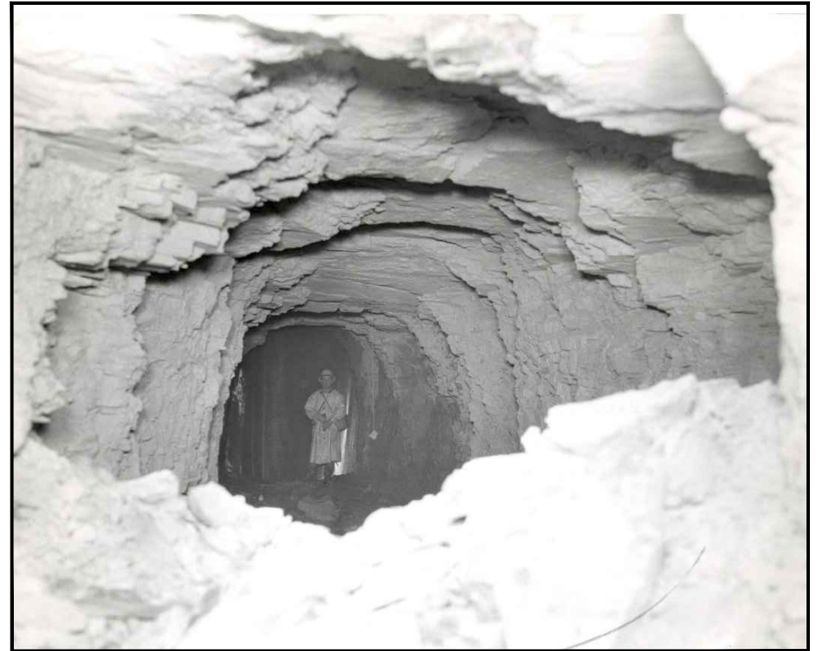
TYPICAL DEEP TUNNEL INTERCEPTOR CONSTRUCTION. NOTE UNSUPPORTED ROOF WITH HORIZONTAL CROWN BREAK. CONTRACT AND LOCATION UNDOCUMENTED.
