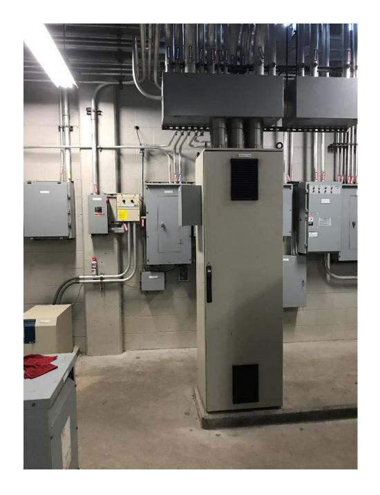
LPB 001 – 709 to power effluent channel equipment
