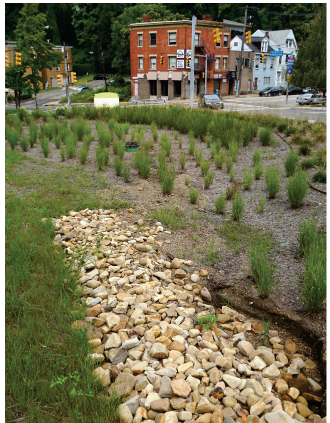
Completed June 2018 by the Pittsburgh Water and Sewer Authority, this stormwater infrastructure project at Centre and Herron in the Hill District was partially funded by ALCOSAN's GROW program and will manage approximately one million gallons of runoff annually.
