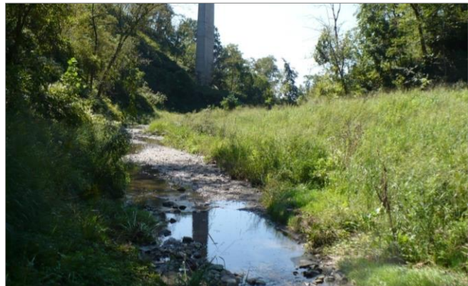
Figure 10-75: Jack’s Run stream was re-routed out of the combined sewer system and restored
