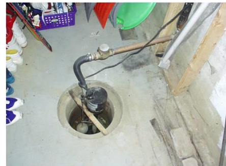
Figure 10-74: Sump pump disconnection from sanitary sewer
