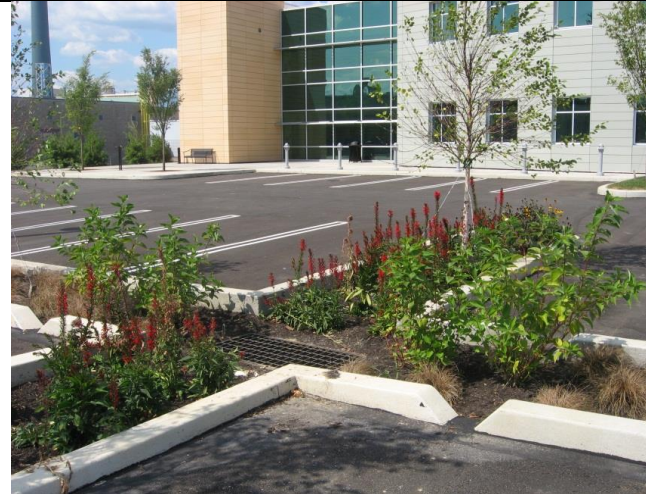
Figure 10-8: GSI Redevelopment Example: ALCOSAN Customer Service Building
