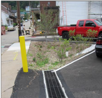
Figure 10-42: Etna Borough GSI Installation at Walnut and School Street
