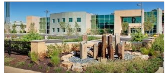
Figure 10-79: ALCOSAN's CS&T Building parking lot uses a rain garden and bio-swale to capture and infiltrate stormwater
