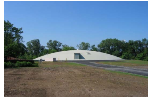
Example Aboveground /Below Ground Storage Tank for Possible SSO/CSO Control Onondaga County, NY
