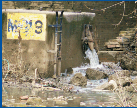
A Combined Sewer Overflow (CSO) occurs when stormwater and sewage, carried in a single pipe, overload the sewer system and flow untreated into rivers and streams. CSOs contain a variety of pollutants such as debris, chemicals, bacteria, and animal waste.
