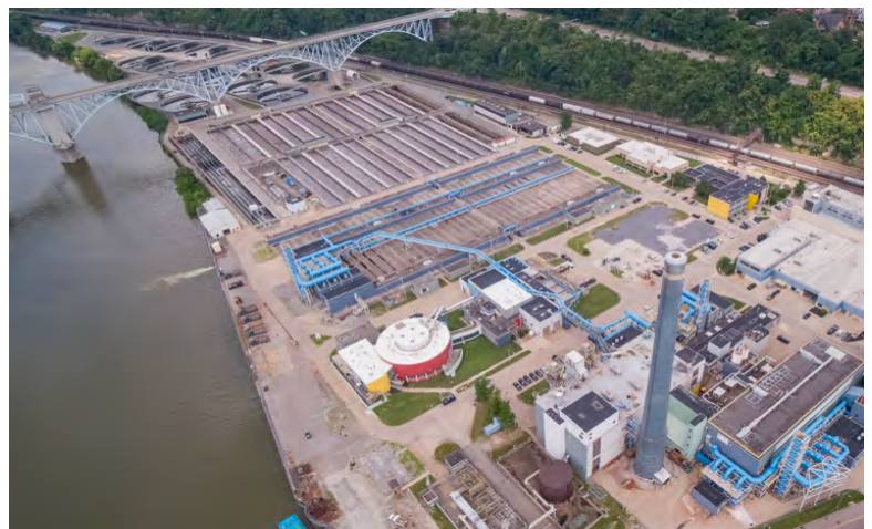
Aerial photographs show the 60-year evolution of ALCOSAN's wastewater treatment plant from 1959 (top) to today.
