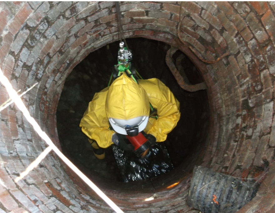
A Regional Conveyance employee inspects flow monitoring equipment
